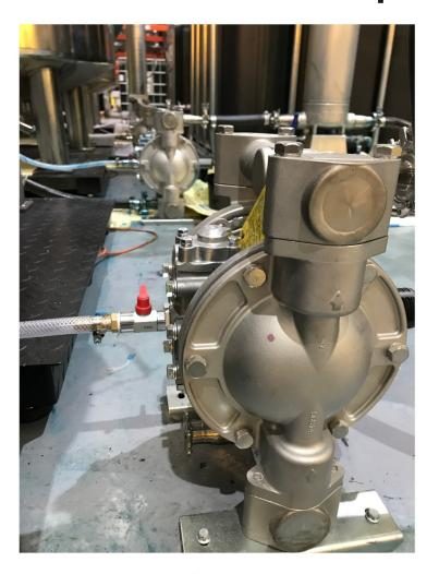
In total, we specified and supplied 25 of Yamada's clean operating AODD pumps. Some for raw ingredient additions to process and the remainder for transfer of the finished product from the mixers to IBC holding tanks.
