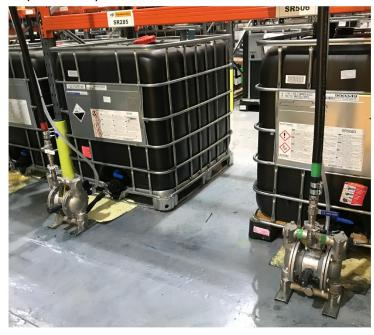
As the distributor for Yamada pumps in the UK, we opted for an air operated double diaphragm (AODD) pump in stainless steel construction and PTFE internals.
