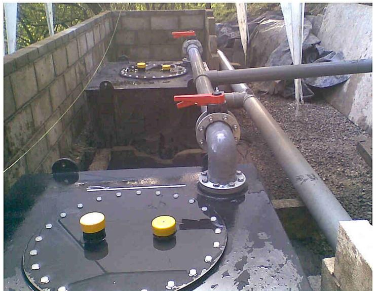
Access hatches, sparge pipes, manifolds and fill chambers were also built and upgraded. The associated filtration and UV sterilisation system was then upgraded for the client to complete the project.
