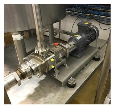
Our solution was to turn to Fristam Pumps and their FDS twin screw range. Such was their product confidence, Fristam offered a trial pump. This allowed us to demonstrate a selected pumps capability to draw syrup directly from a room temperature tank and pump up 3m to production.
